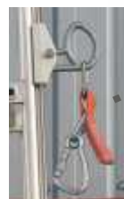
Detail of anti-fall device
